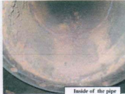
Inside of the pipe
