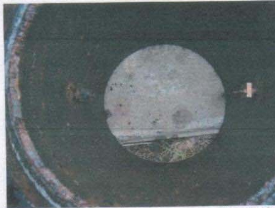
Fig.(11): Visual inspection of the Corrosion coupon ( to the left) and scale coupon (to the right)
