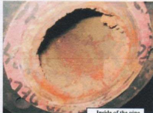
Inside of the pipe
